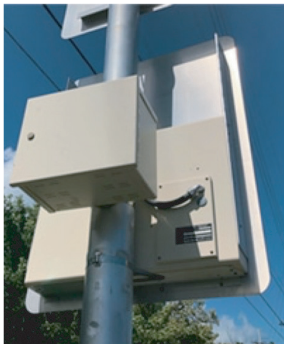
Most common LED Signage Installation
